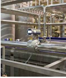
FLOW MEASUREMENT OF DEMINERALIZED WATER
