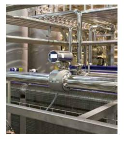
FLOW MEASUREMENT OF DEMINERALIZED WATER
